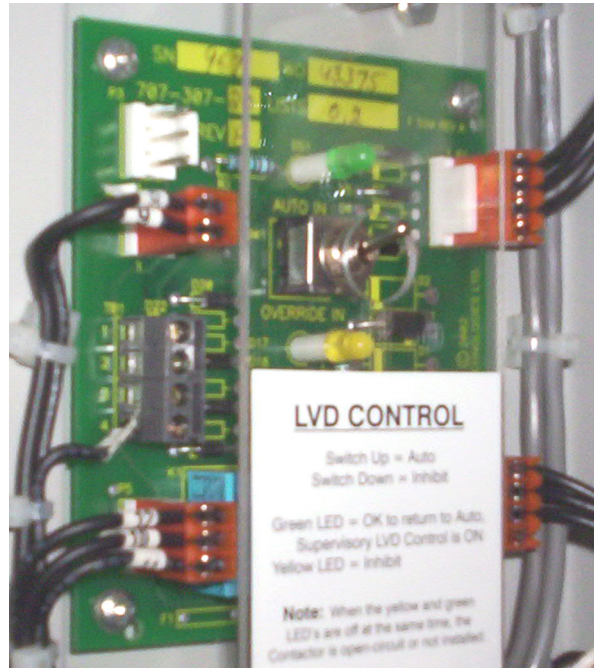
Figure 8 — LVD override control and distribution alarm card
