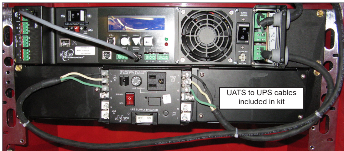
Figure 14 — FXM 350 UPS AC Power Connection Wiring from UATS
