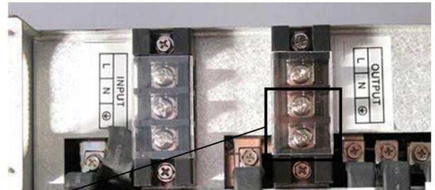
4. Connect AC input to the terminal on the back left of MBSDU panel according to the position of the labels as shown.
