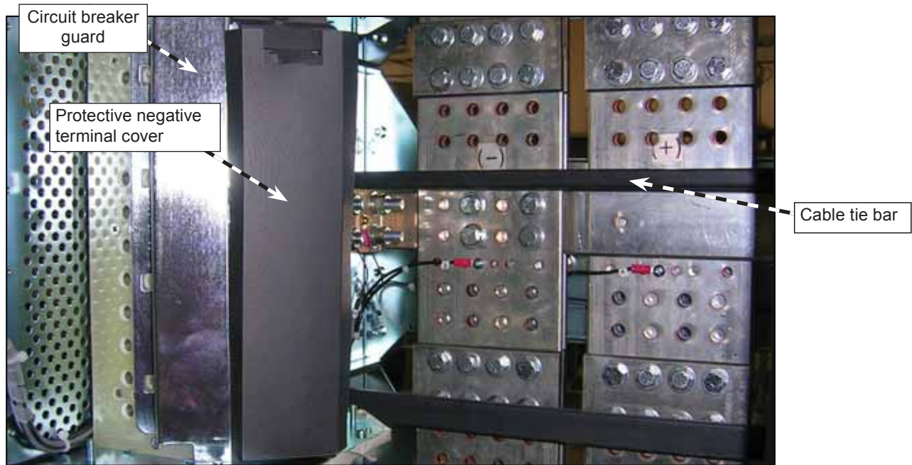
Figure 36 — Breaker distribution module before load cables are installed
