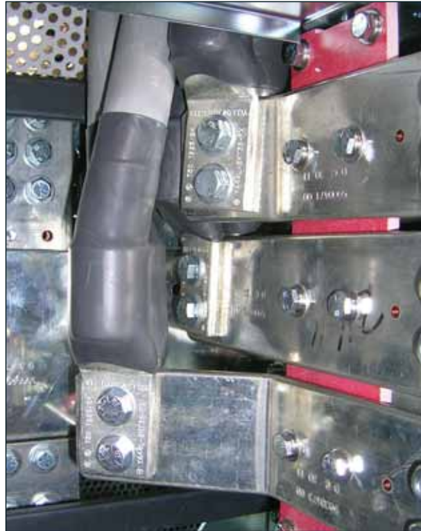
Figure 38 — High capacity TPL fuse wiring (shown with 2x 750 MCM wire)
