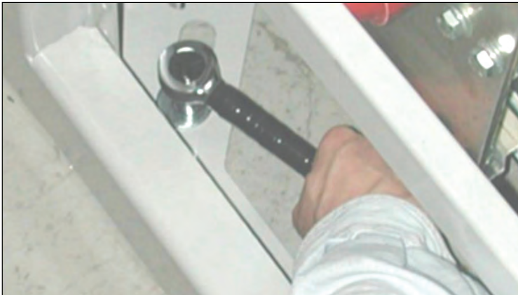
Figure 6 — Securing power system bay to concrete floor
