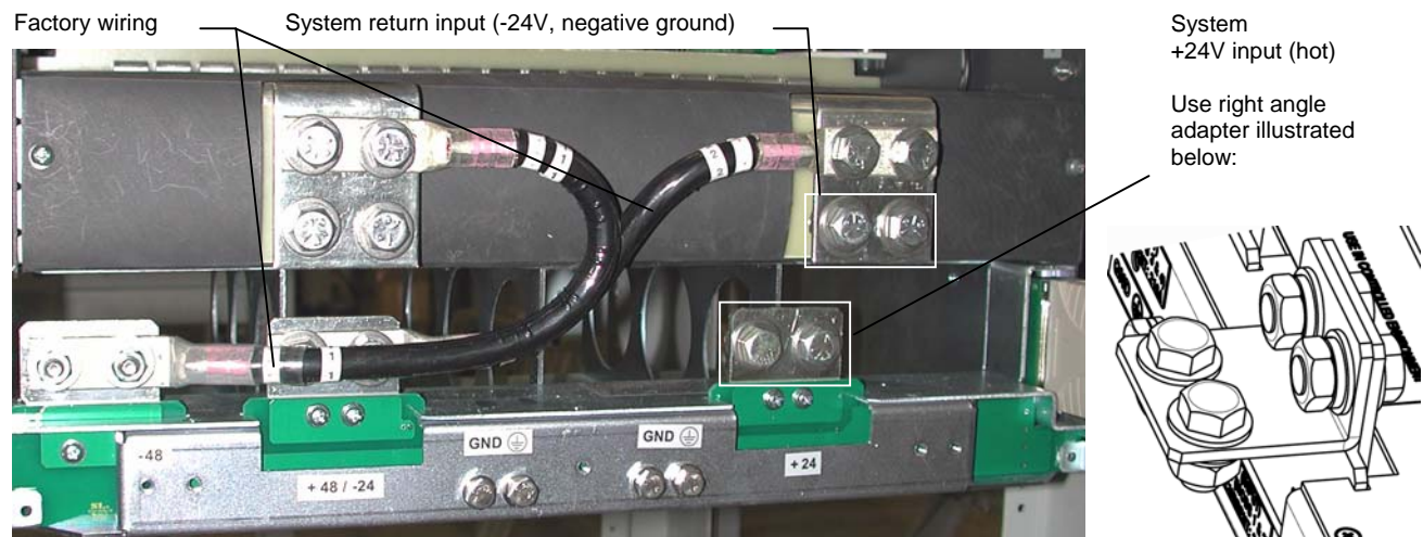
Figure 9—Rear view of CXPS 24-48-i showing factory wiring, input (and return) to system
