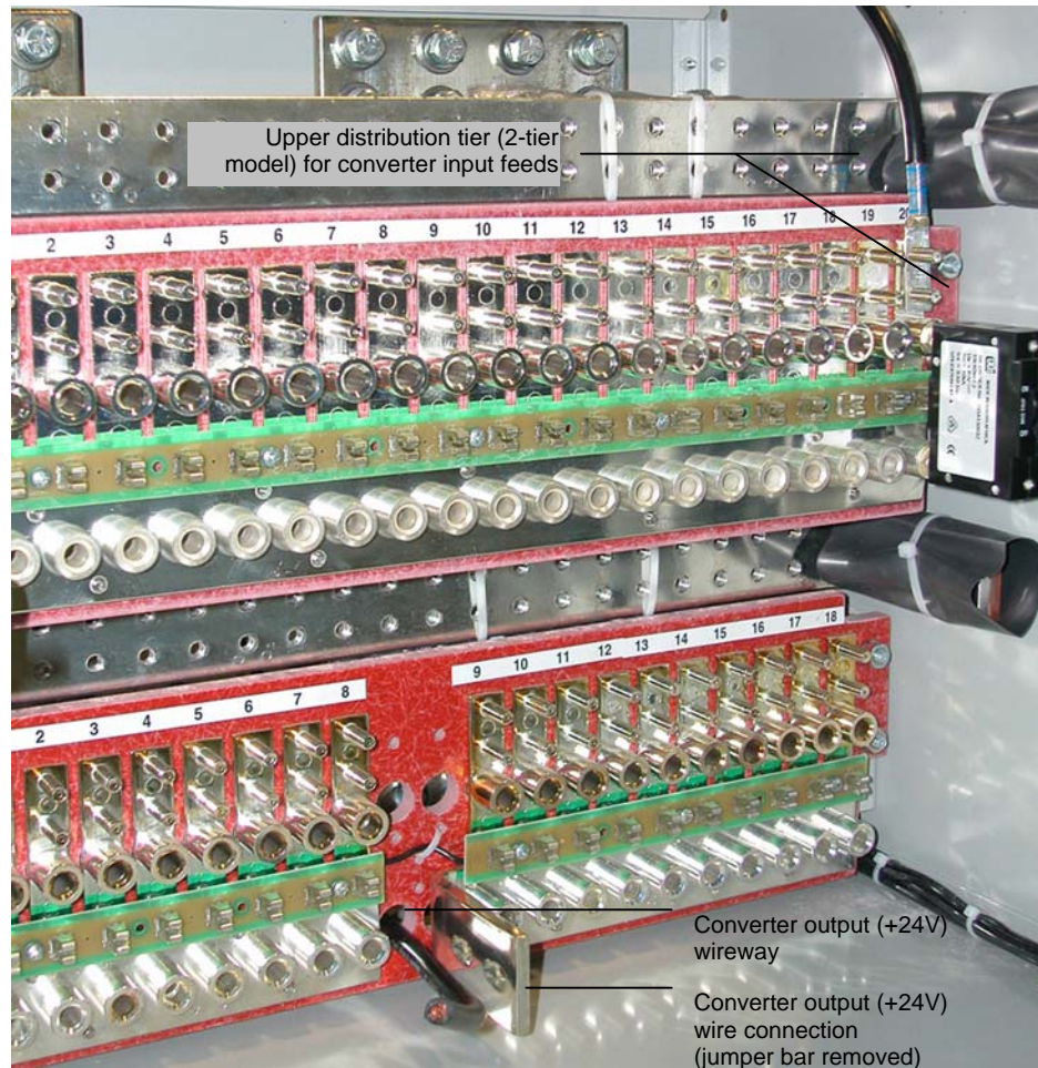
Figure 12–Connection points and wire routing for +24V input into split tier distribution
