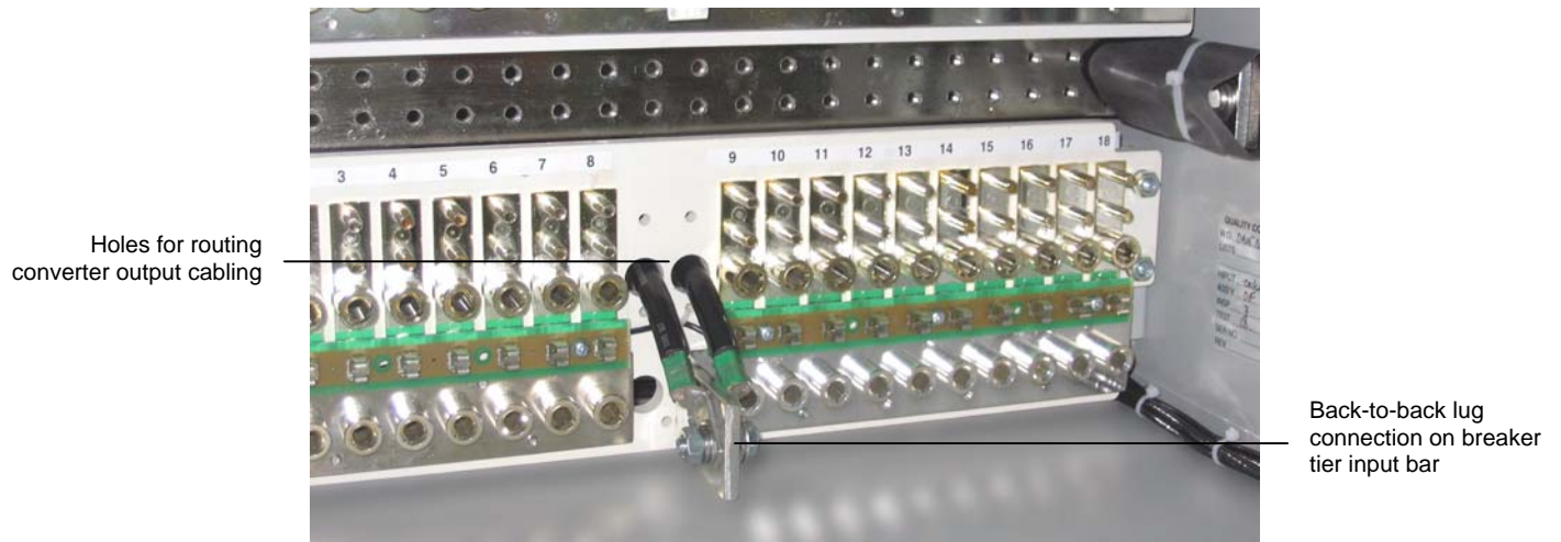
Figure 15—Converter output (48Vdc) connection to distribution tier
