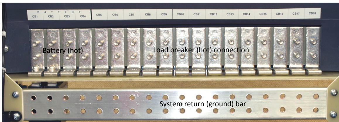
Figure 10–Battery, load, and return connection locations
