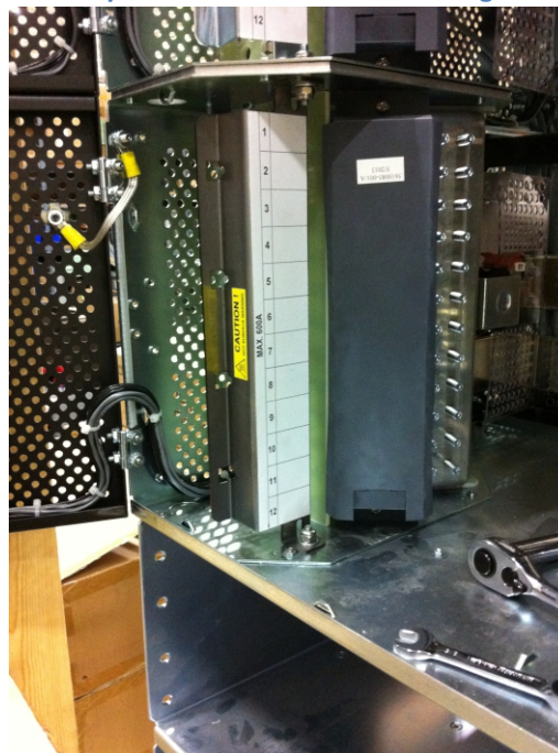
Figure 7: Installed New Guard Should Swing Freely
