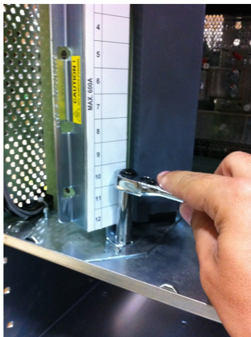
Figure 2: Remove Nylock nuts
