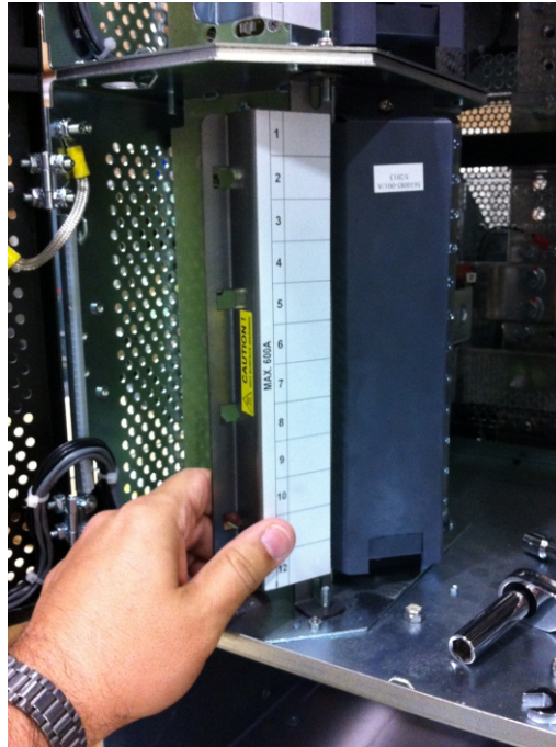
Figure 3: Discard Old Guard & Replace w/New Guard
