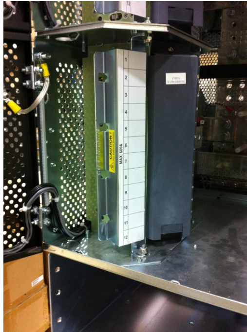
Figure 1: Locate the Older CB Guards within the CXDM
