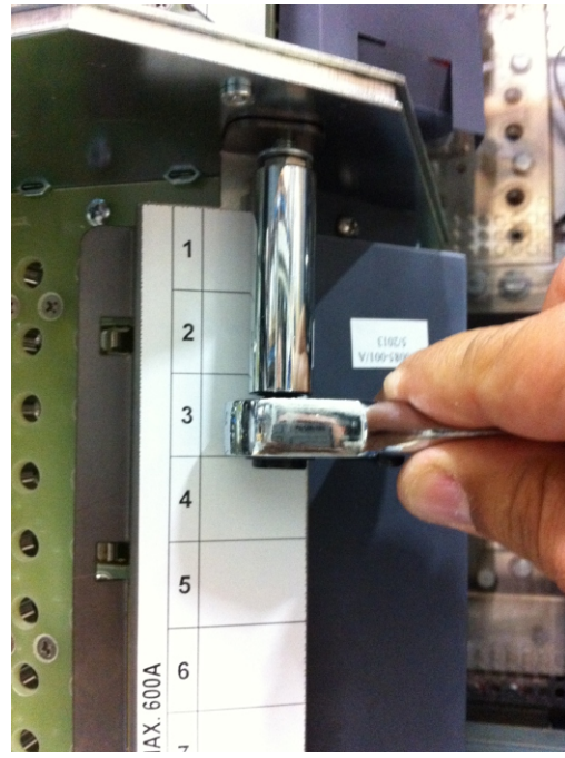
Figure 6: Tighten Top Nylock Nut
