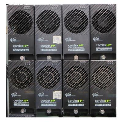
4.6. CXCM4 controller replacement with a rectifier module procedure is completed.
