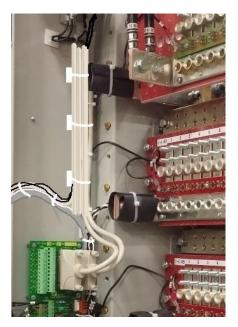
3.12. Route Shunt cable and CAN cable from bottom of the distribution.
