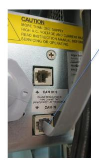
CAN cable from L-ADIO on a Single Rectifier Shelf system.
