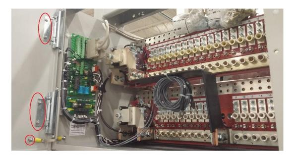
1.2 Remove the lock from the existing door and install in new door.
