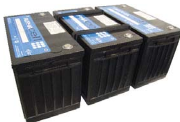
Recommended 36V Battery string spacing utilizes two clips
