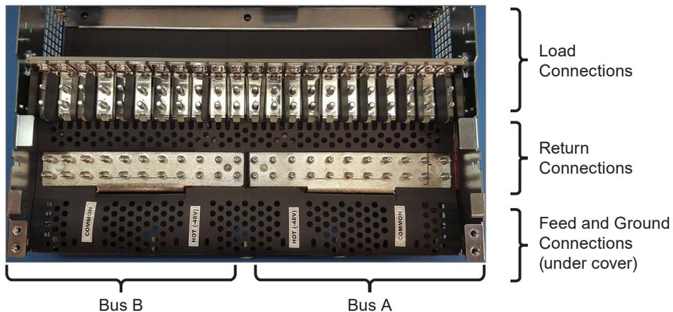
Figure 3 — Feed Connections
