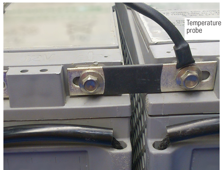
Figure 47: Battery temperature probes, battery bay
