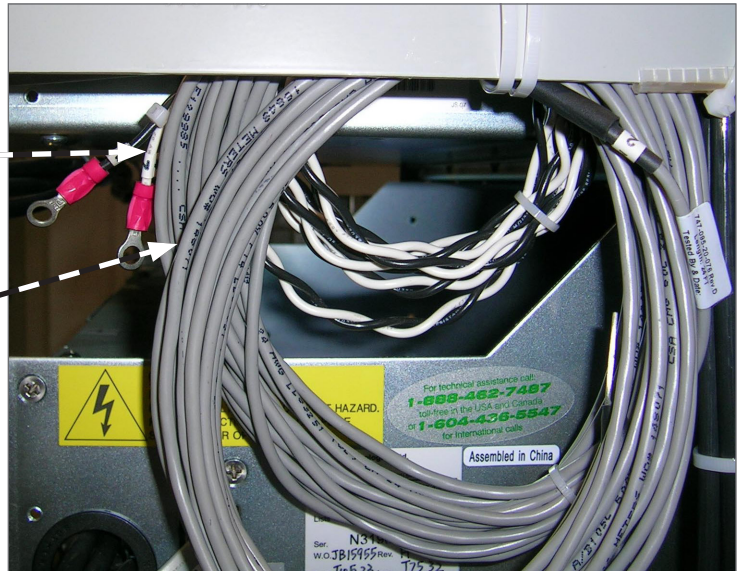
Figure 32: Shunt and interbay signal cables
