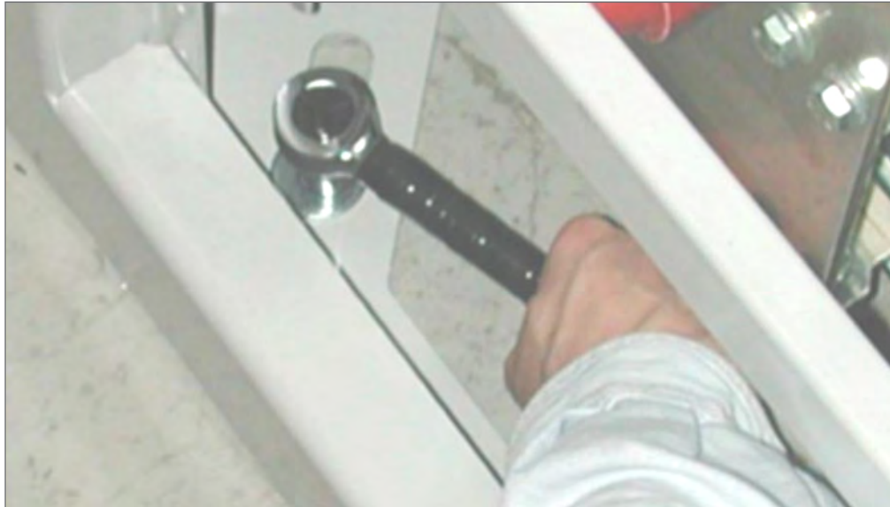
Figure 26: Securing power system to concrete floor
