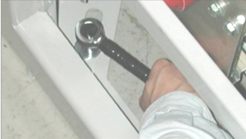
Figure 27: Securing power system to concrete floor
