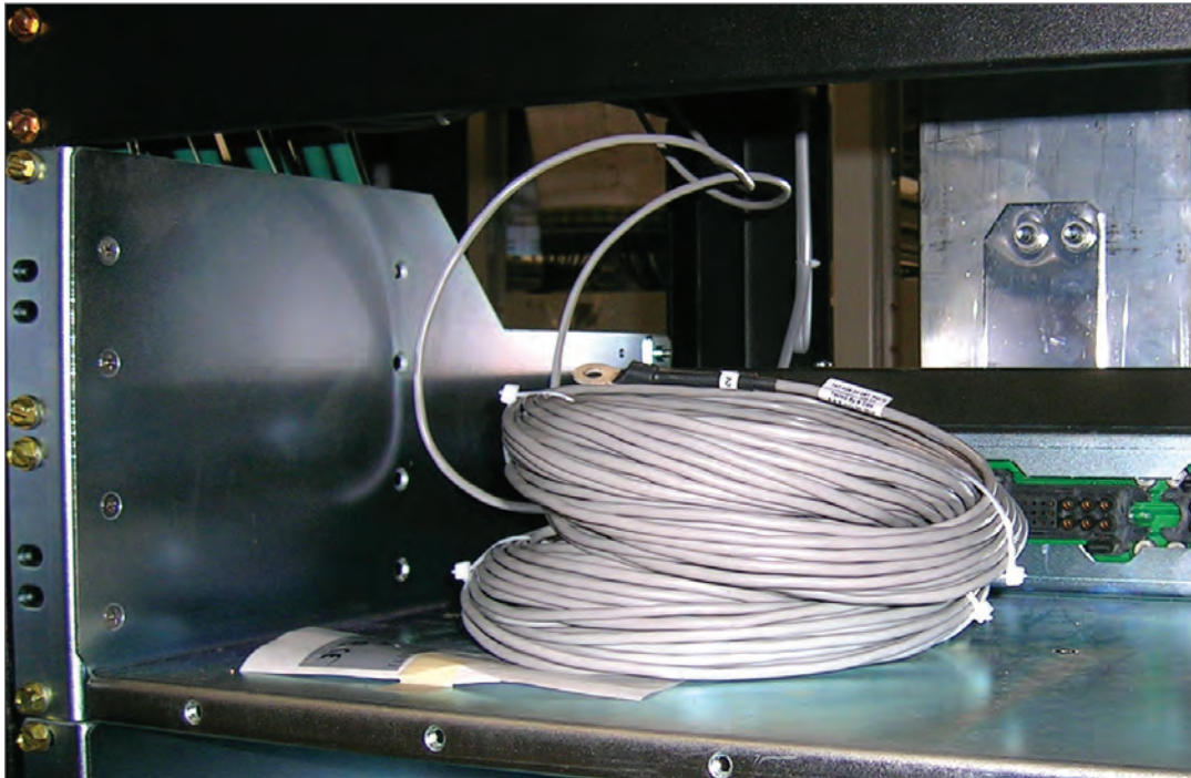
Figure 31: Battery temperature probes
