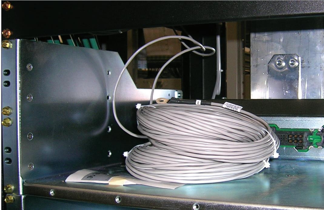
Figure 32: Battery temperature probes
