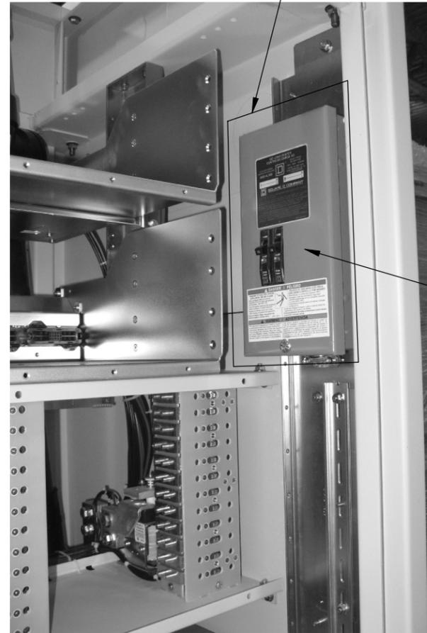
Te41 AC LOADCENTER AIR CONDITIONER AC POWER CONNECTION FROM Te40
