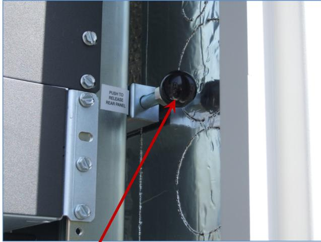
Push on knob to release rear slam latch panel.
