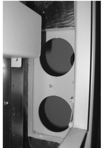
REMOVE TOP CORNER KNOCKOUTS ON FACING SIDES OF BOTH ENCLOSURES (2 PER SIDE) TO ACCEPT BOLTING HARDWARE
