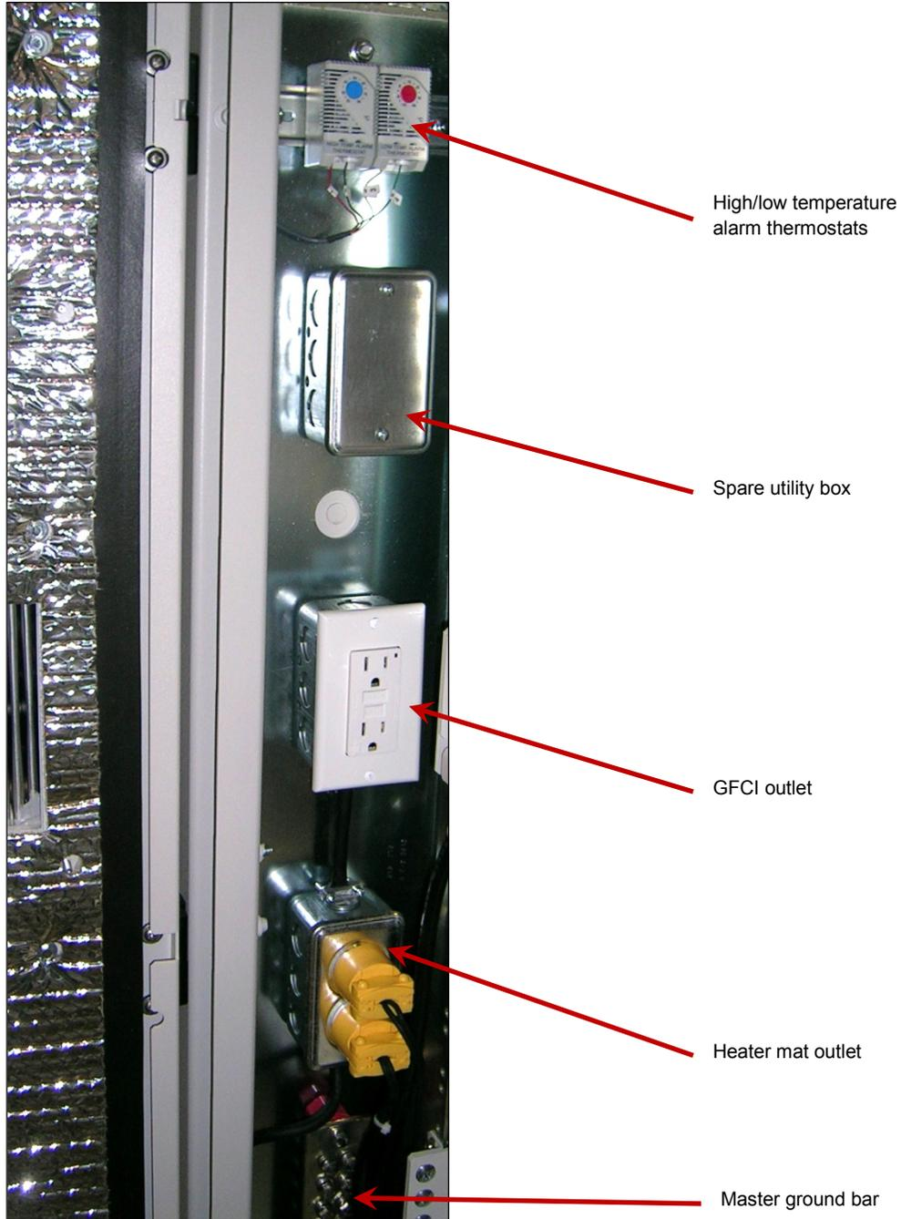
Figure 2 - Miscellaneous compartment features
