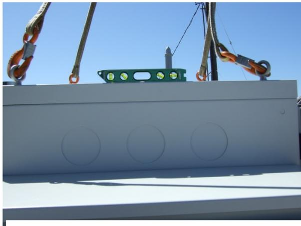
**Figure 14 - Secure hooks in eyebolts**
