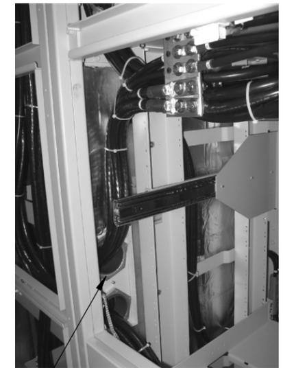
NEATLY ROUTE CABLES THROUGH BOTH CHASE NIPPLE FITTINGS. PUT NEGATIVE CABLES THROUGH TOP NIPPLE AND POSITIVE CABLES THROUGH BOTTOM NIPPLE TO KEEP CABLES ORGANIZED.
