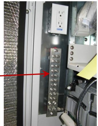
**Figure 15 - Enclosure ground connections**
