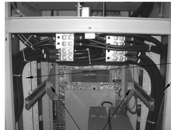
KEEP ALL INTERFACE CABLES AWAY FROM REAR SECTION OF EQUIPMENT SLIDES. USE CABLE TIES PROVIDED TO ATTACH INTERFACE CABLES TO SIDES OF EQUIPMENT RACK CHANNELS AS NECESSARY.
