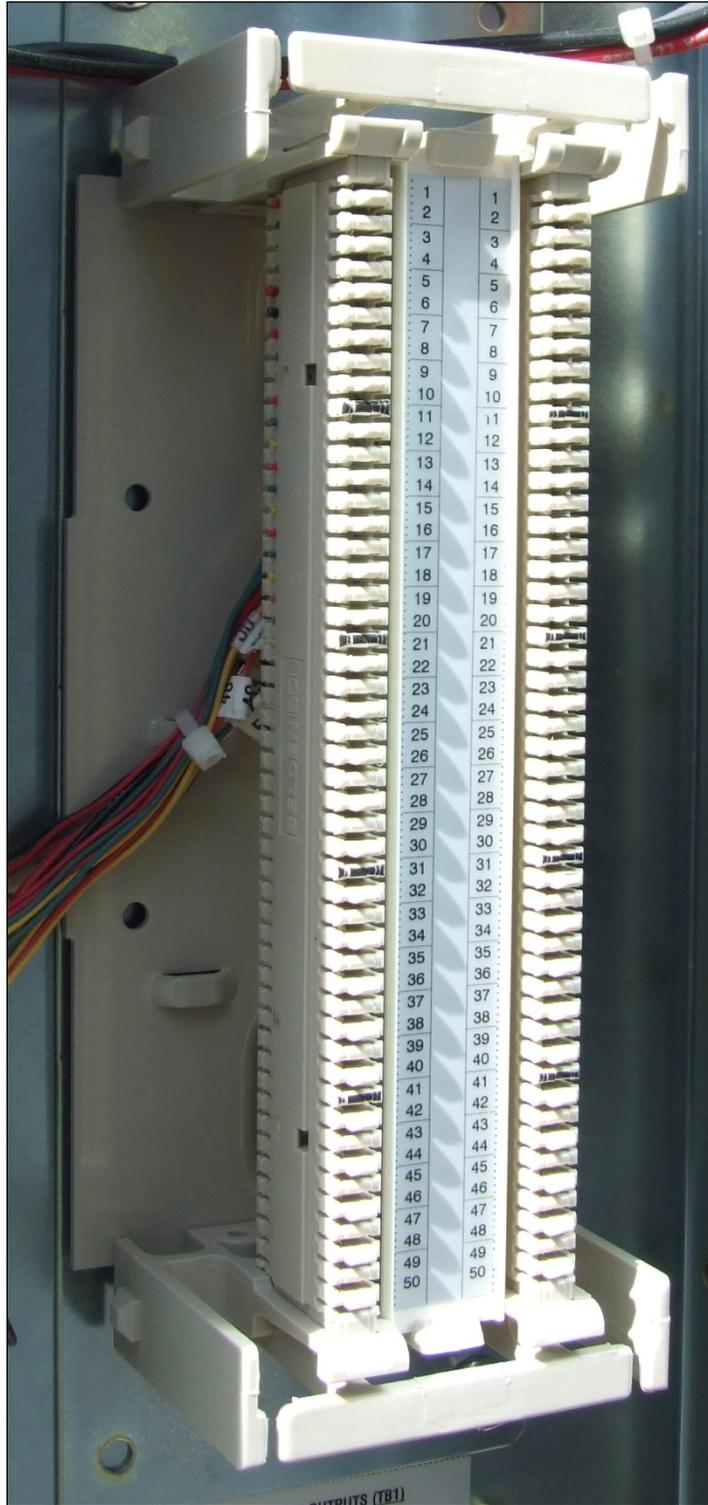
**Figure 4 - Alarm "Bix" block**
