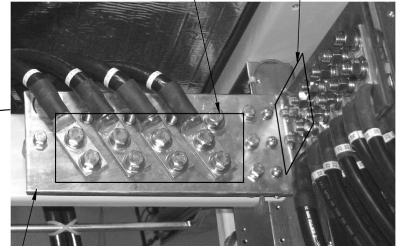
OBSERVE PROPER BUS POLARITY ON THIS SIDE!
