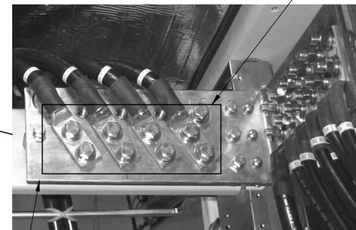
OBSERVE PROPER BUS POLARITY ON THIS SIDE!
