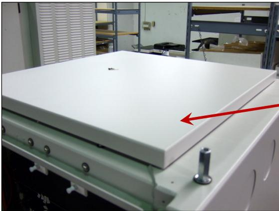
Remove solar shield exposing hatch plate.
