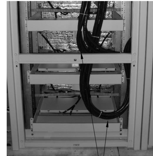
DRAPE INTERFACE CABLES DOWN FROM CABLE TIE-OFF BAR. USE CABLE TIES PROVIDED TO NEATLY DRESS/BUNDLE CABLES TOGETHER.
