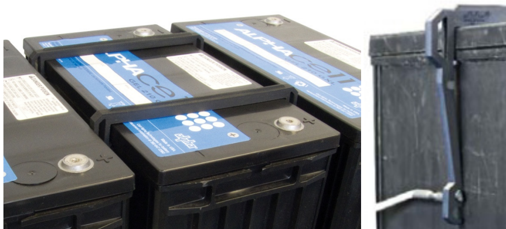
Figure 5 – BSC spaced out the batteries and secured BTS
