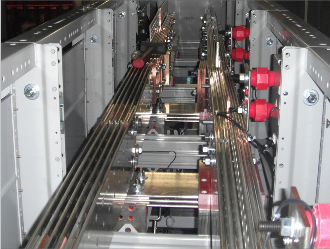
Figure 33 — Example of Installed Inter-bay Buswork
