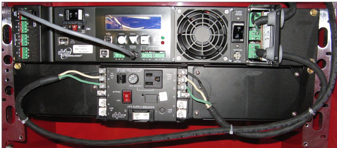
Figure 16 — FXM 350 UPS AC Power Connection Wiring from UATS
