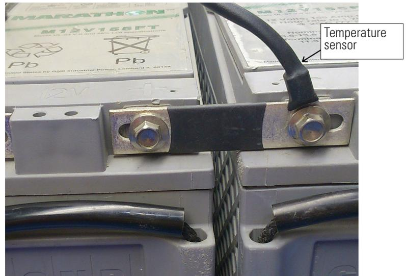
Figure 29: Battery temperature sensor, battery bay
