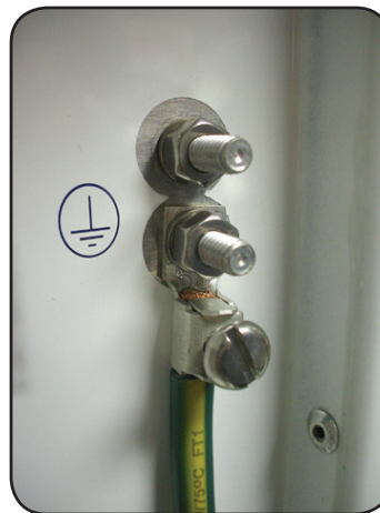
Figure 6.17 - Protective Earthing Terminal
