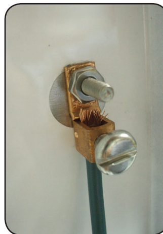
Figure 6.18 - Grounding the UPS
